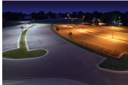
Figure 3.23 LED vs. HPS lights [33]
